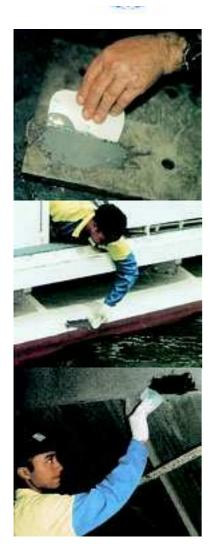
FAST STEEL PUTTY Fast curing steel putty that enables emergency repairs to be carried out with minimal down time. Cures at very low temperature to a tough inert material that can be machined, drilled or tapped. Repair production critical equipment such as valves, tanks, pipes and other components quickly to minimise downtime in plant and processing applications.
